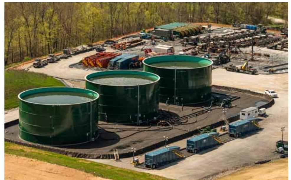
A diverse approach to water treatment means: removal of suspended solids, inorganic scale forming compounds, petroleum hydrocarbons/organics, and friction reducers and other polymer additives. In addition to this, sterilization is achieved and water is treated to the operator’s desired specification.
